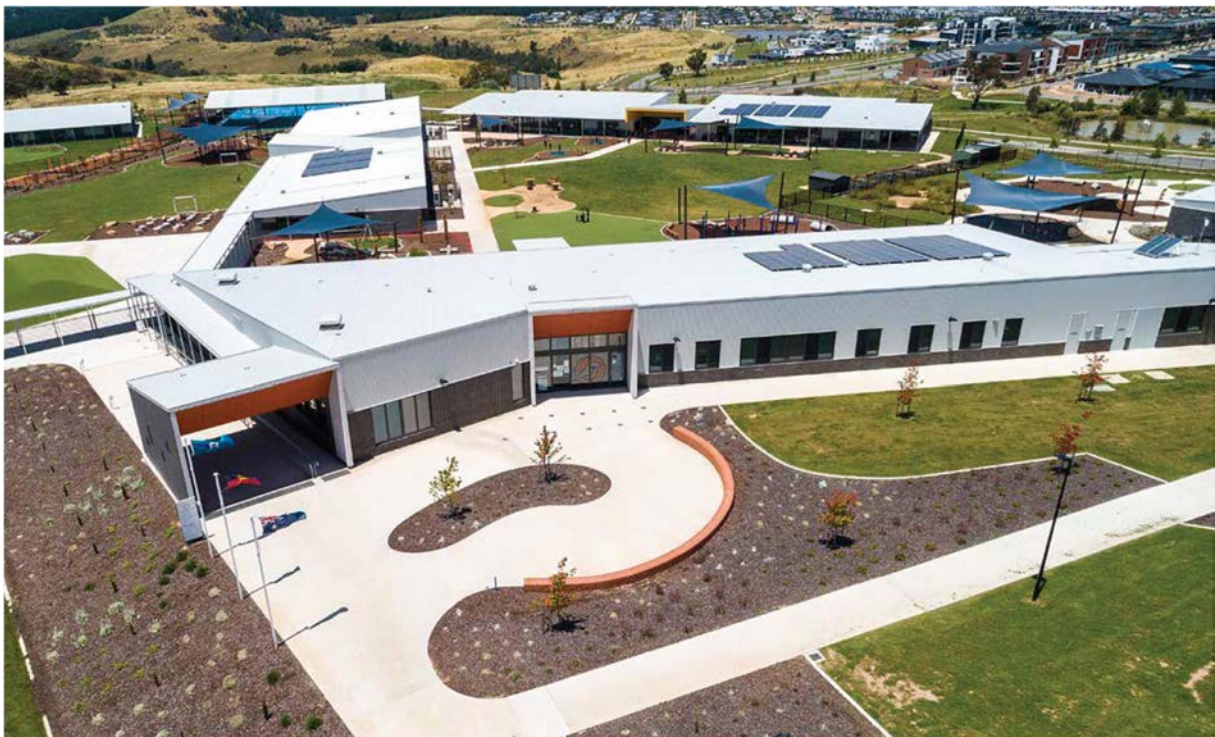
Evelyn Scott School Solar Panels
