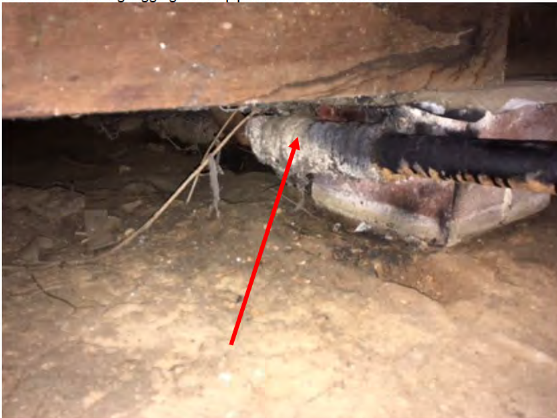
Areas of remaining lagging where pipes leave removal area
