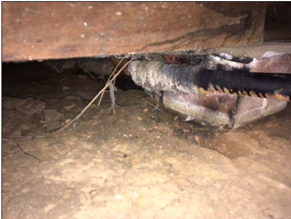
Visible lagging after black painting and before pink PVA glue spraying
