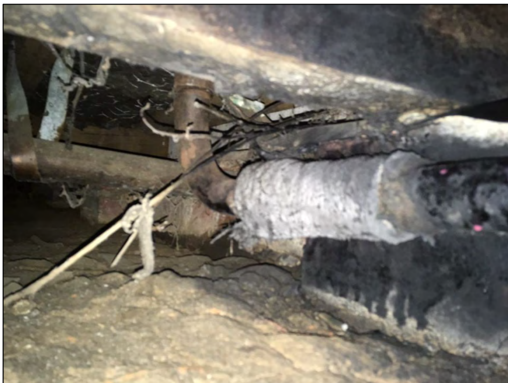
Visible lagging after black painting and after pink PVA glue spraying
