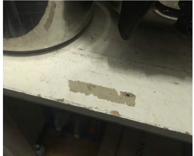
Figure 4: Pantry bench top – area where paint has flaked chipped or been worn away
