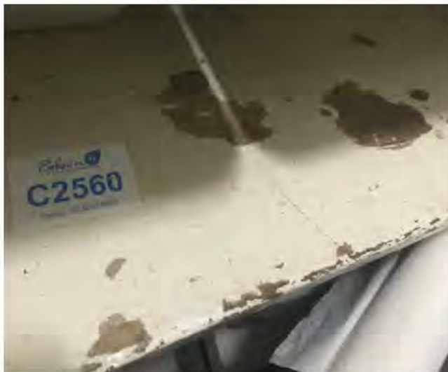
Figure 1: Pantry bench top – areas where paint has flaked chipped or worn away
