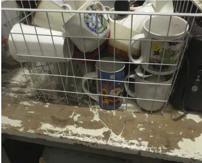
Figure 3: Pantry bench top – areas where extensive wearing of paint has occurred
