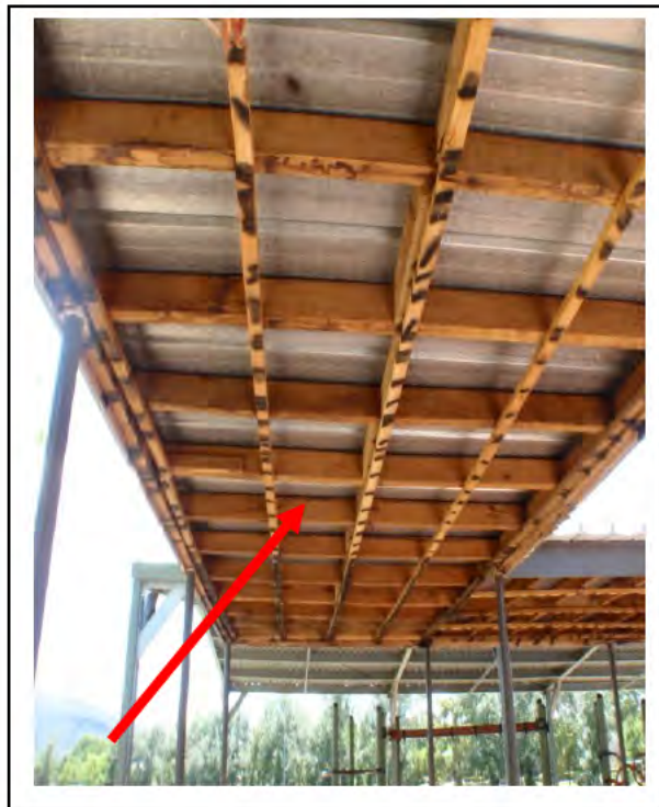
Removal of asbestos soffit sheets from covered walkway from the rear of the main building.
