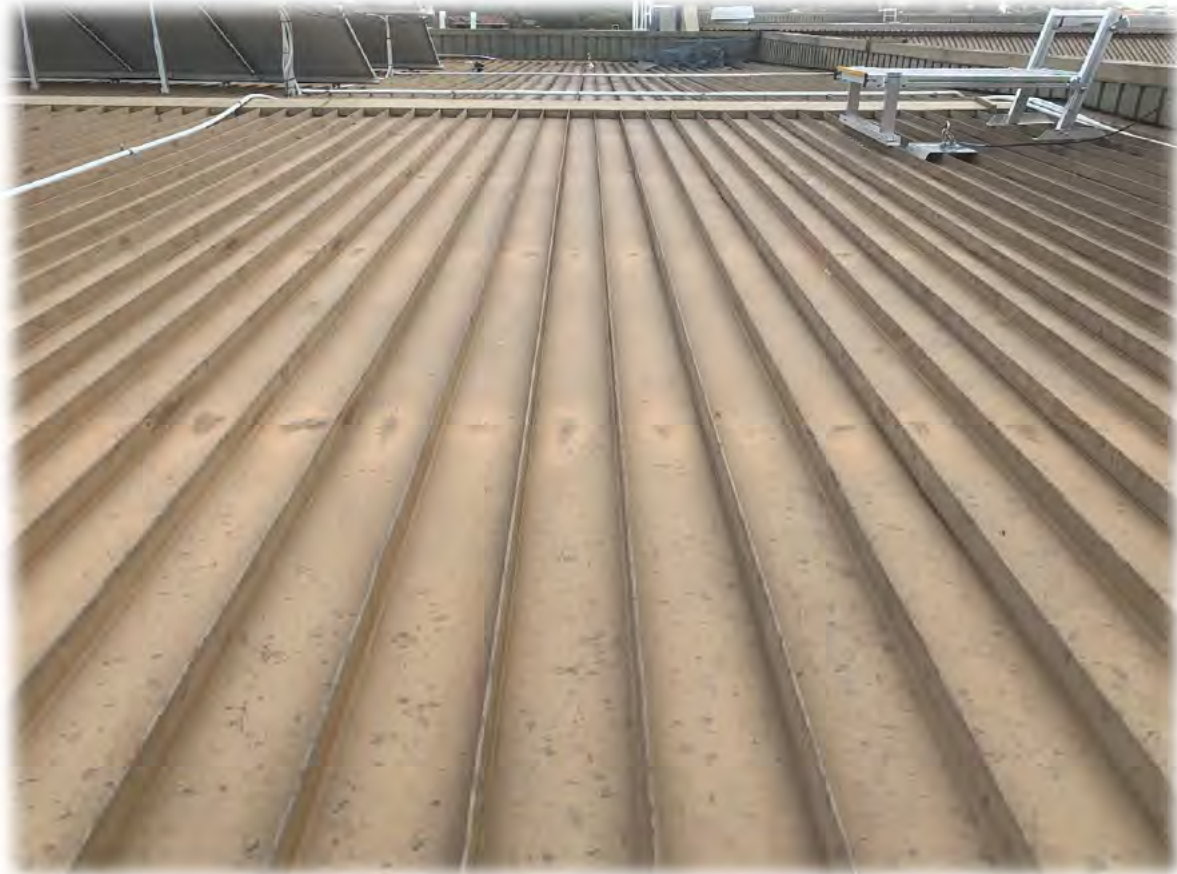
Figure 1: Metal roof cladding
