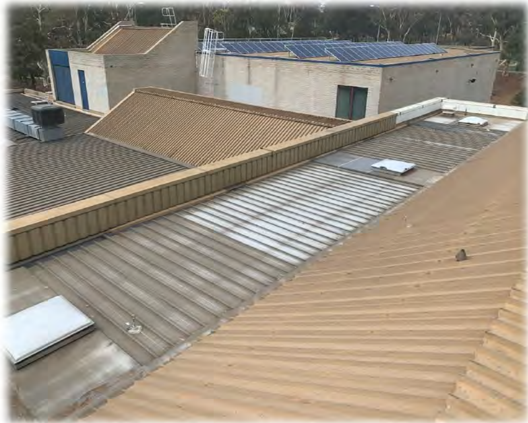
Figure 13: Roof area over dressing and music rooms
