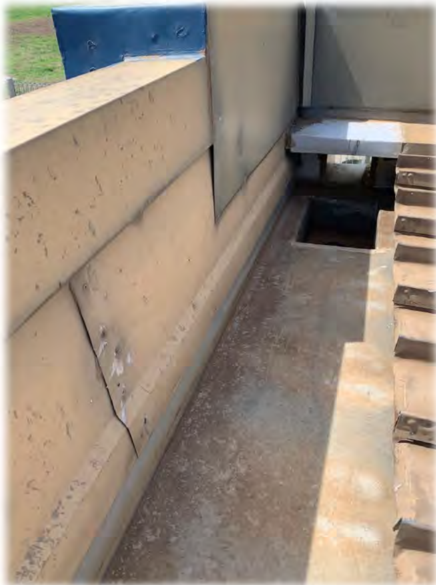
Figure 2: Typical view of box gutter
