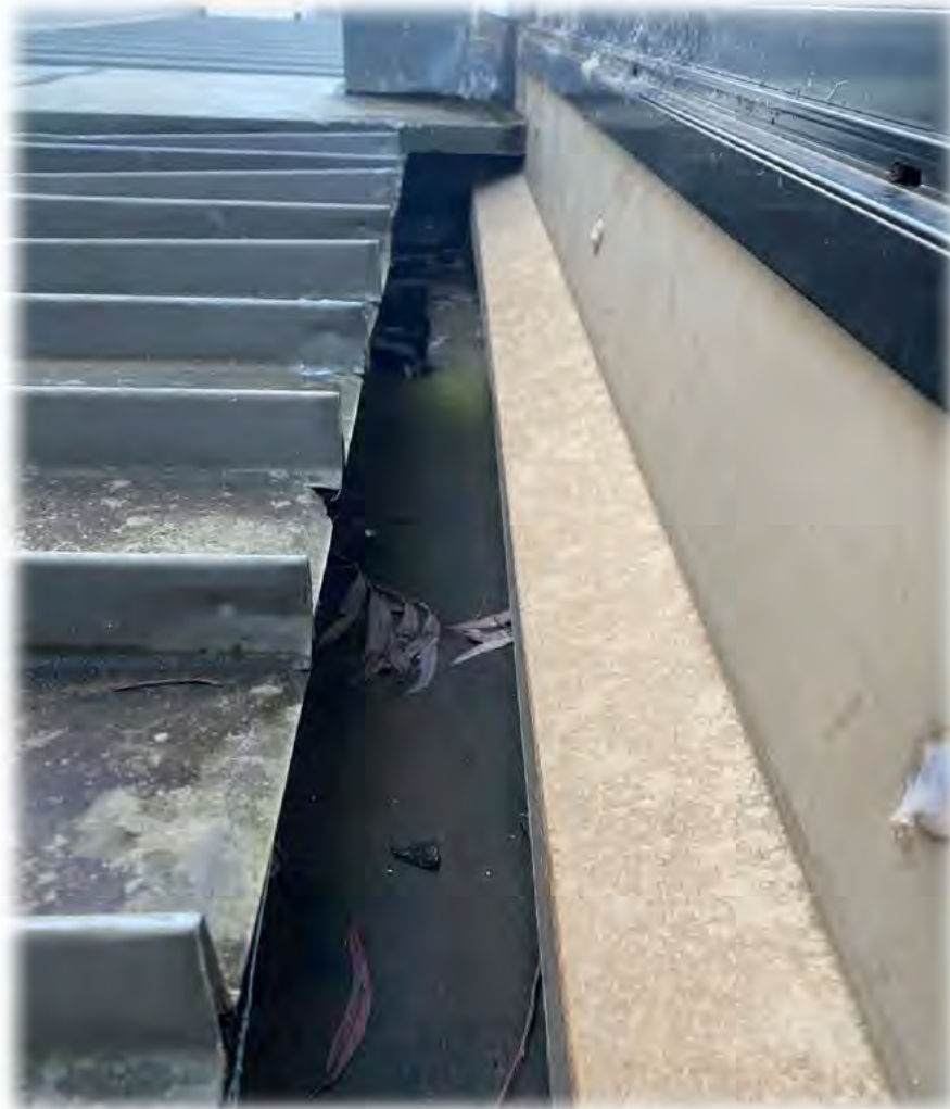
Figure 10: Box gutter located above gymnasium corridor servicing change rooms
