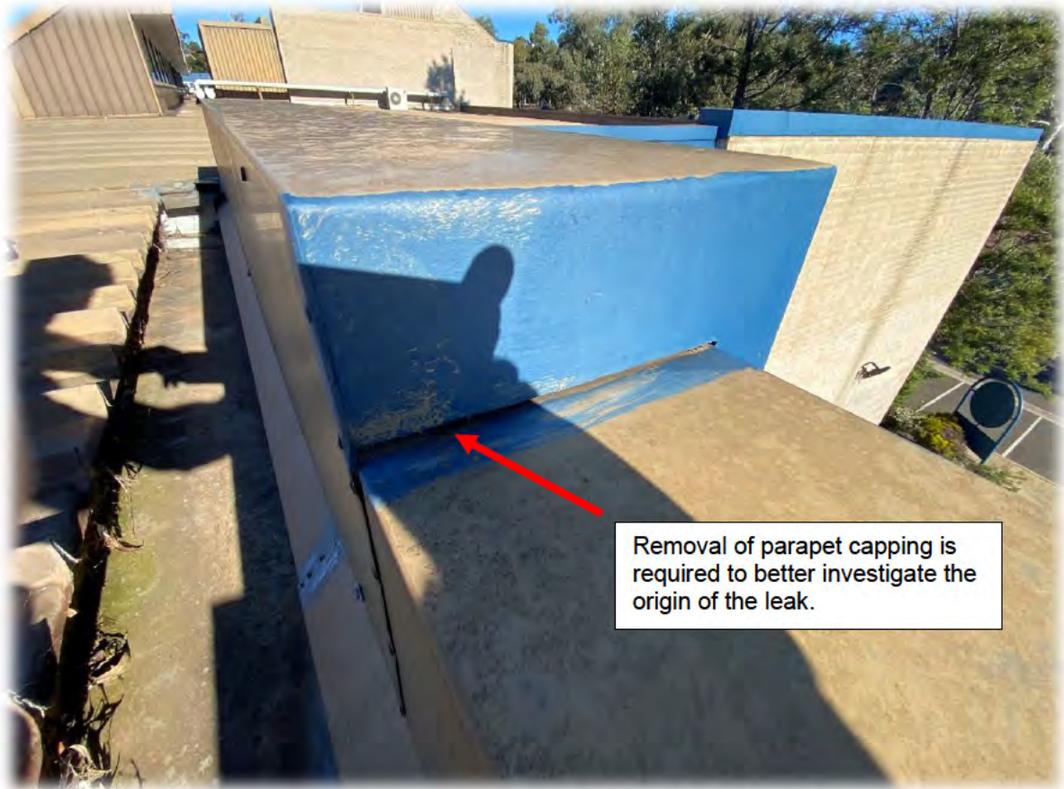
Figure 32: Box gutter and parapet flashing
