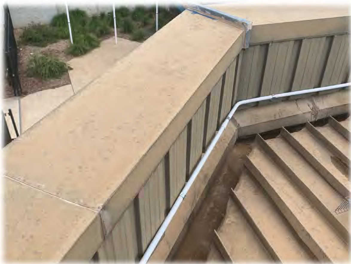
Figure 3: Parapet wall capping and wall and apron flashings
