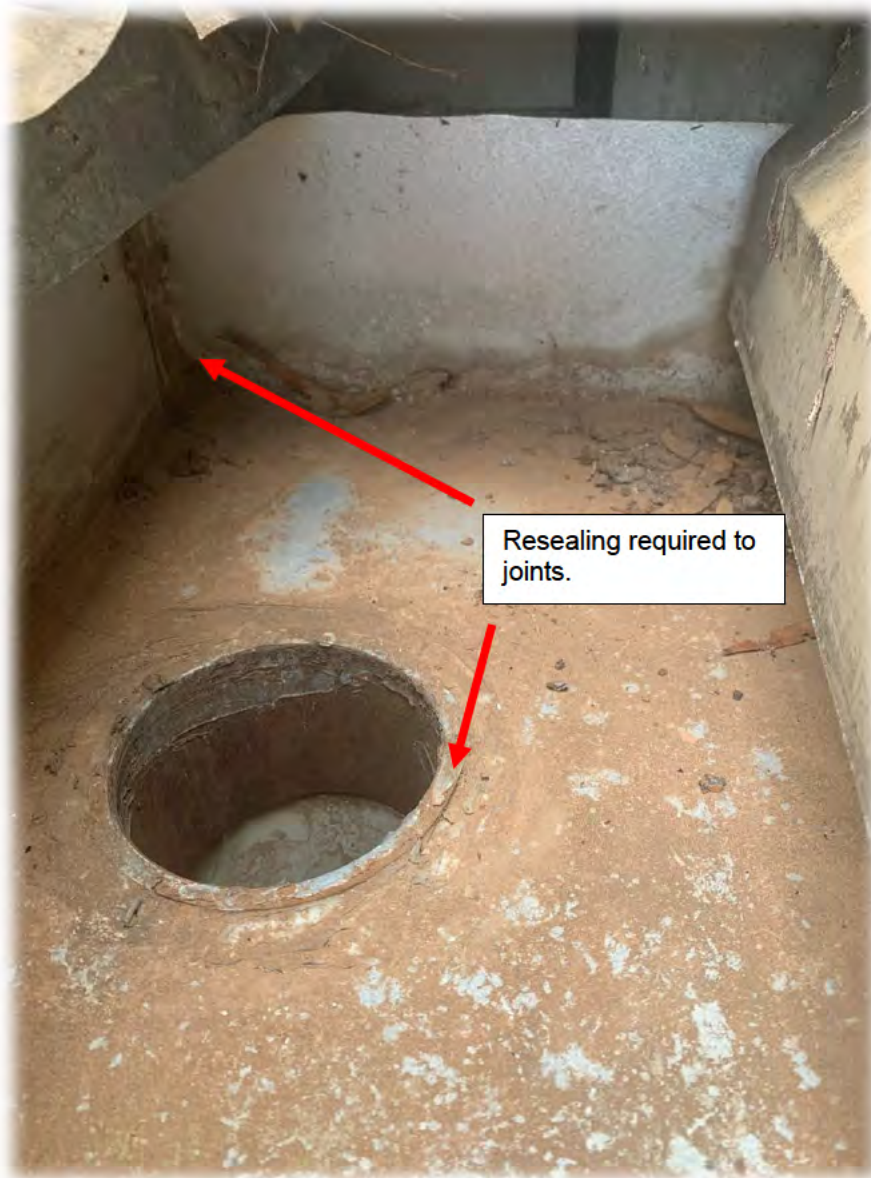
Figure 9: Box gutter outlet
