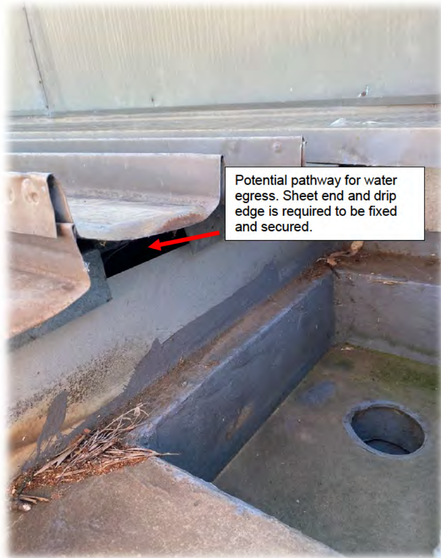
Figure 29: Raised roof sheet
