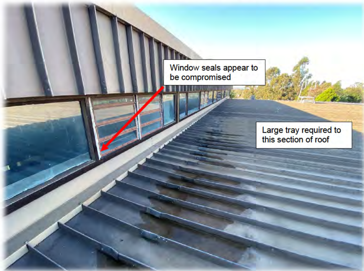
Figure 14: Roof area over library.
