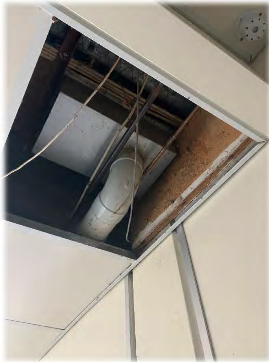
Figure 18: Box gutter sump view from corridor
