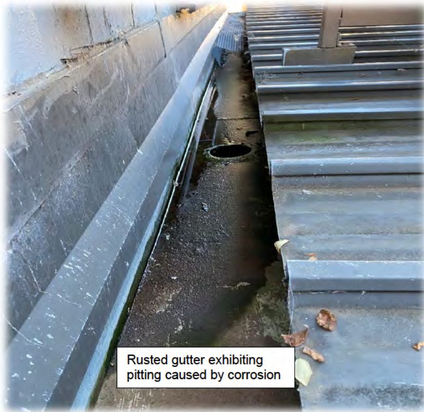
Figure 15: Box gutter along library wall
