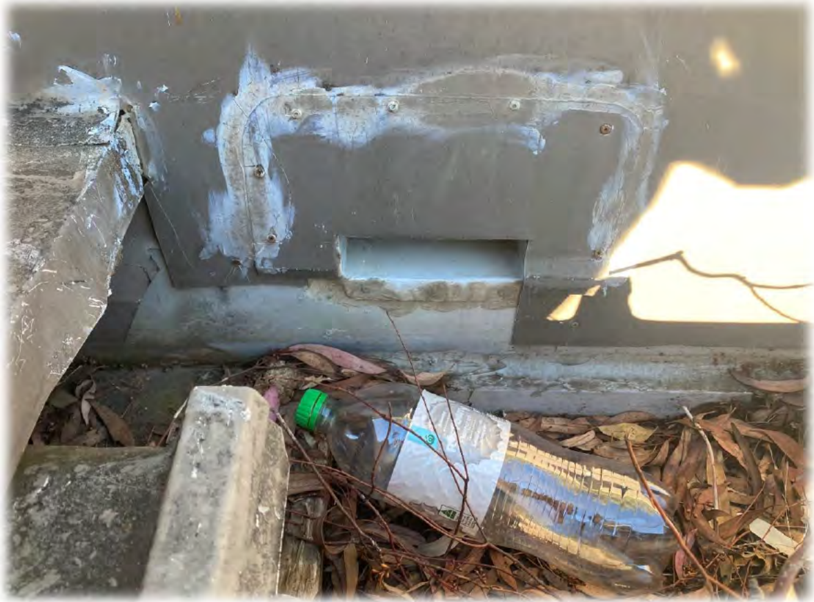
Figure 12: Blocked sump
