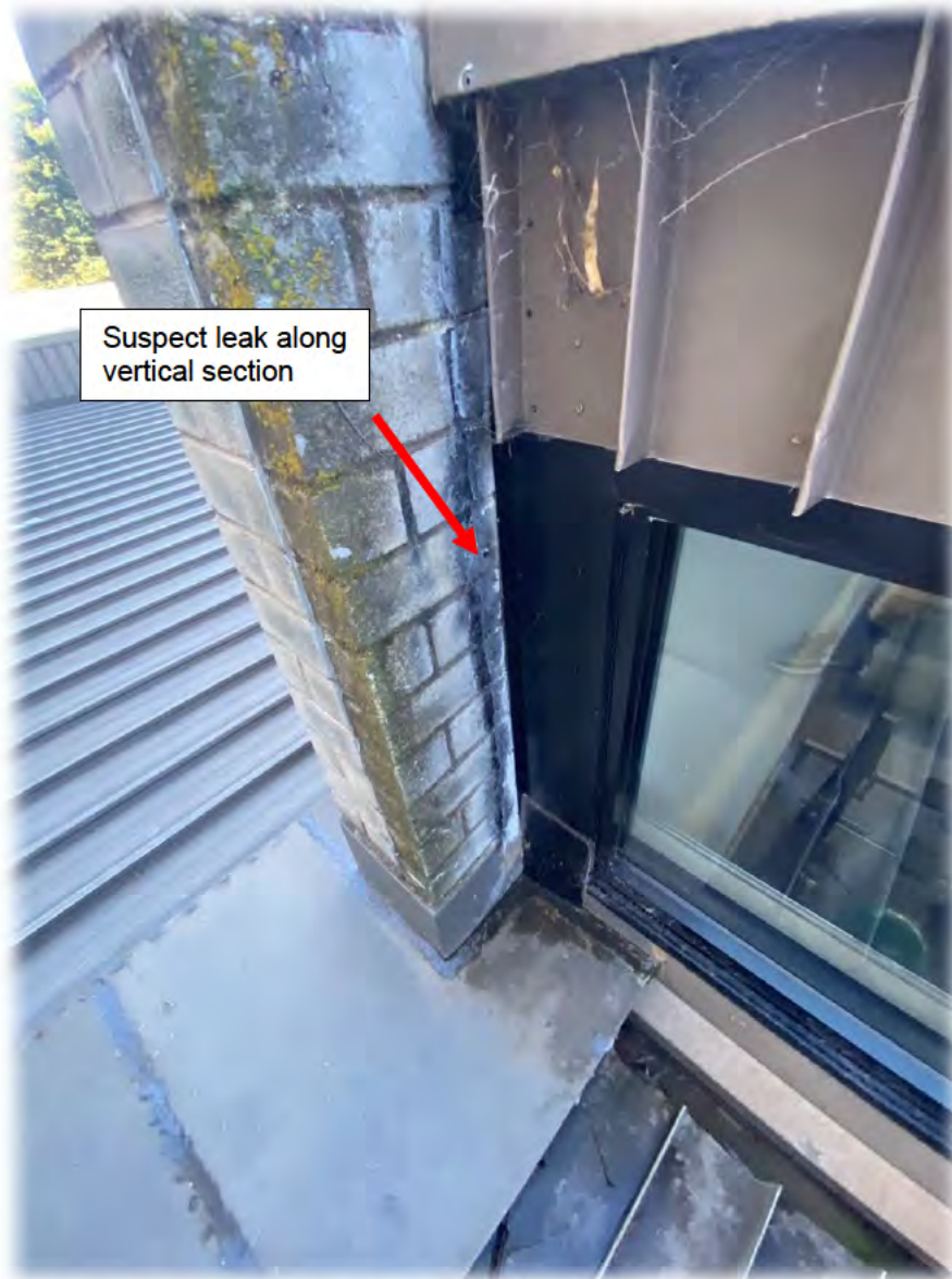
Figure 11: Connecting flashings between newer and original roof cladding over corridor
