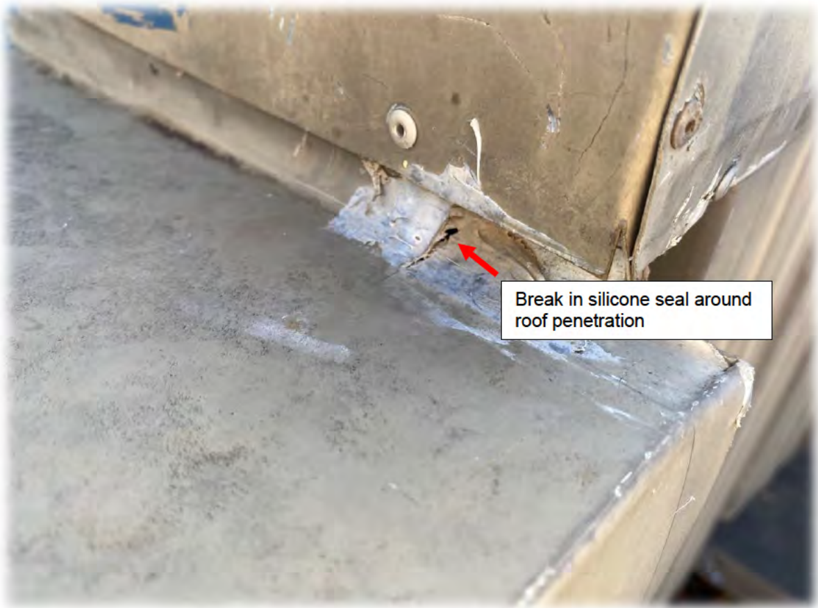
Figure 23: Break in silicone
