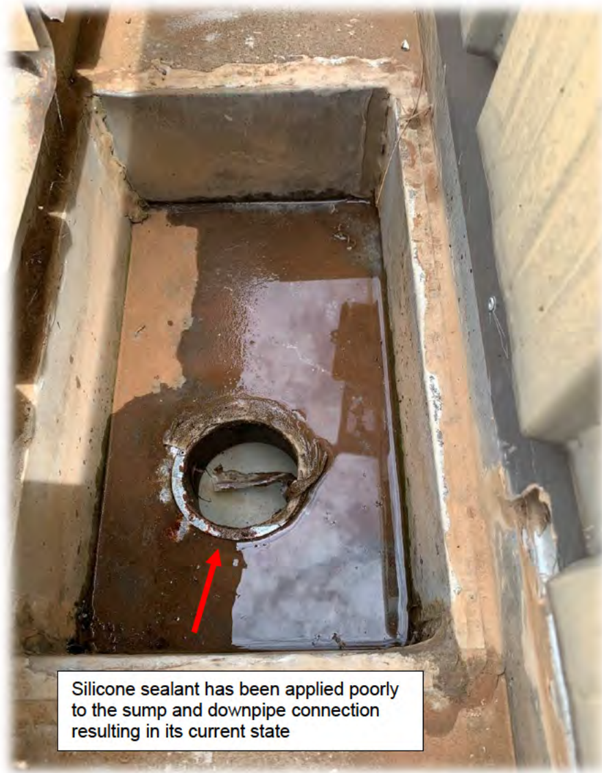
Figure 19: Box gutter and sump
