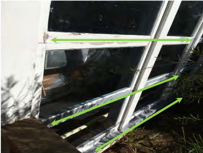
Figure 4: Exterior surfaces after removal of flaking and peeling lead paint
