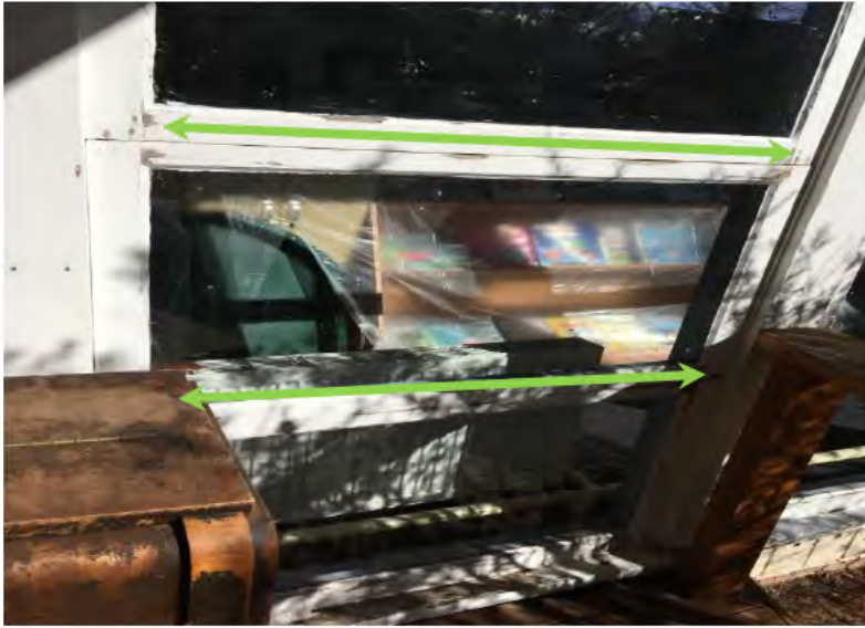
Figure 3 Exterior surfaces after removal of flaking and peeling lead paint
