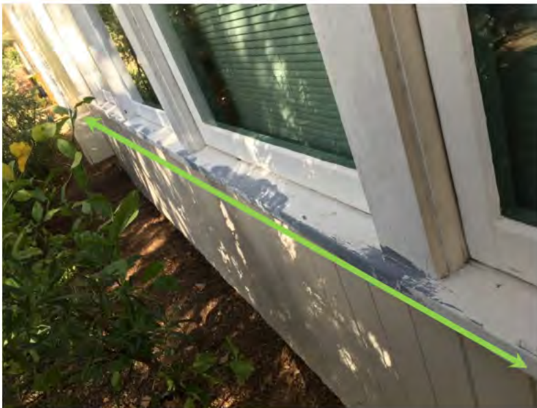
Figure 6: Exterior surfaces after removal of flaking and peeling lead paint
