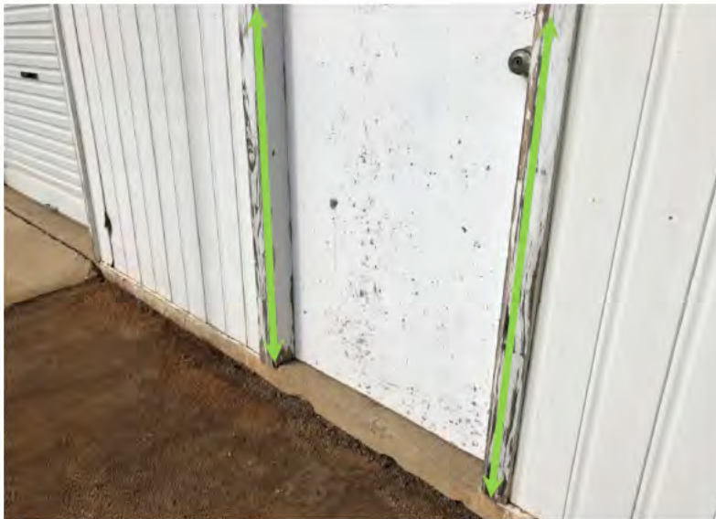
Figure 1: Exterior surfaces after removal of flaking and peeling lead paint
