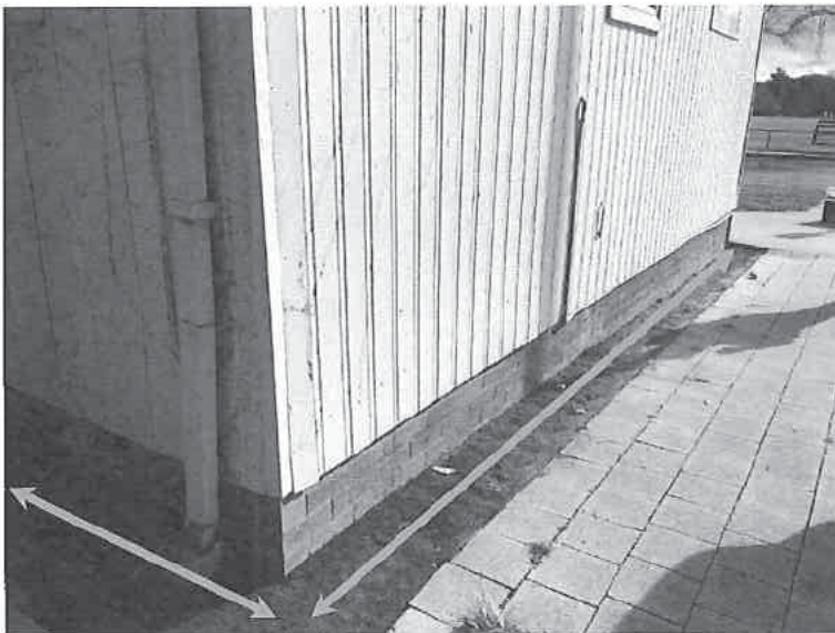
Figure 4: Exterior surrounding soil surfaces after removal of lead paint debris
