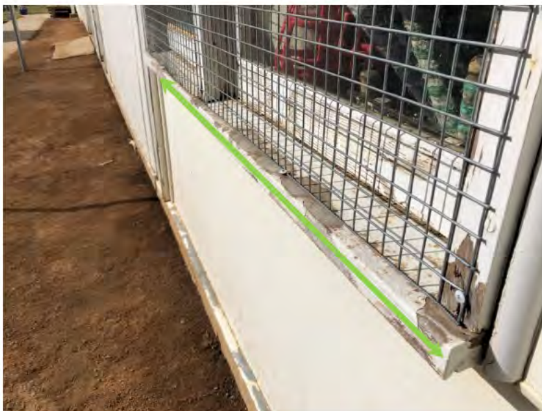
Figure 2: Exterior surfaces after removal of flaking and peeling lead paint
