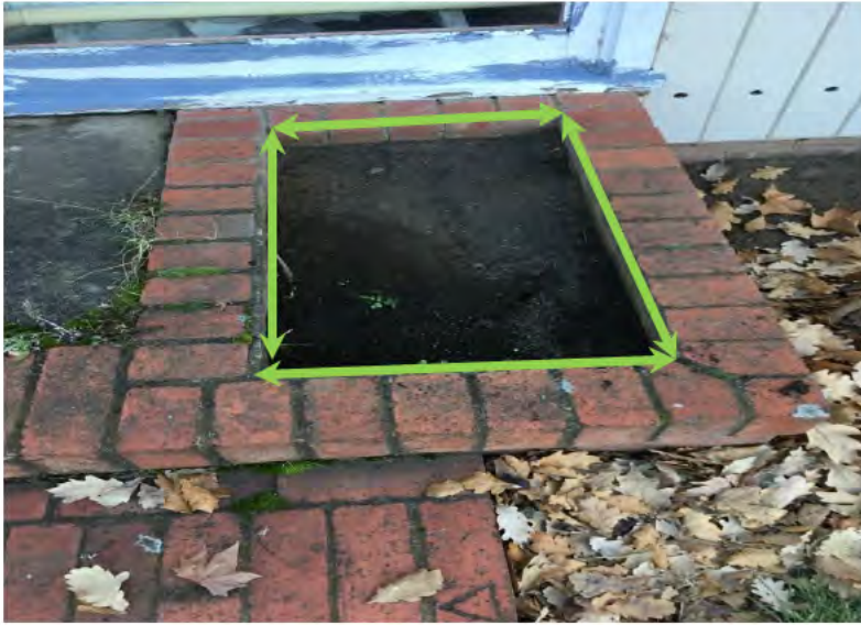
Figure 7: Exterior surrounding soil surfaces after removal of lead paint debris
