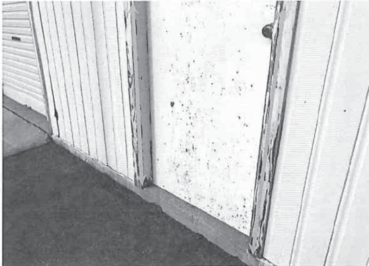
Figure 1: Exterior surfaces after removal of flaking and peeling lead paint
