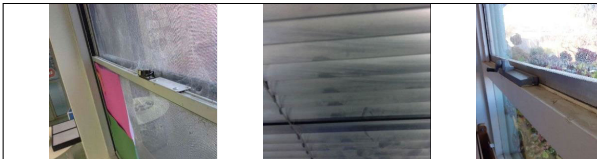
Figure 5: L-R: Cobwebs on interior window Caroline Chisholm Pre-School; Dust on Blinds Caroline Chisholm Pre-School, Dust on sills Curtin Primary
