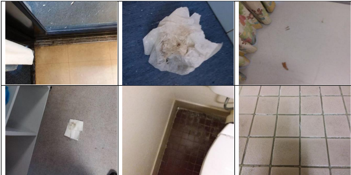
Figure 13: Top L-R: soil build-up on edges and corners (Note soil Buildup on Door track) Malkara; Buildup of grime on vinyl Cranleigh; Floor not swept in classroom Malkara; Bottom L-R: Class room floor Malkara; Toilet cubicle floor Malkara: Toilet flor and grout requires machine scrubbing – Cranleigh
