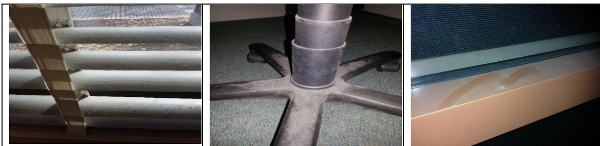
Figure 24: L-R: Dust on Blinds Alfred Deakin High; dust on chair pedestal Hawker high; Dust on sills Belconnen High
