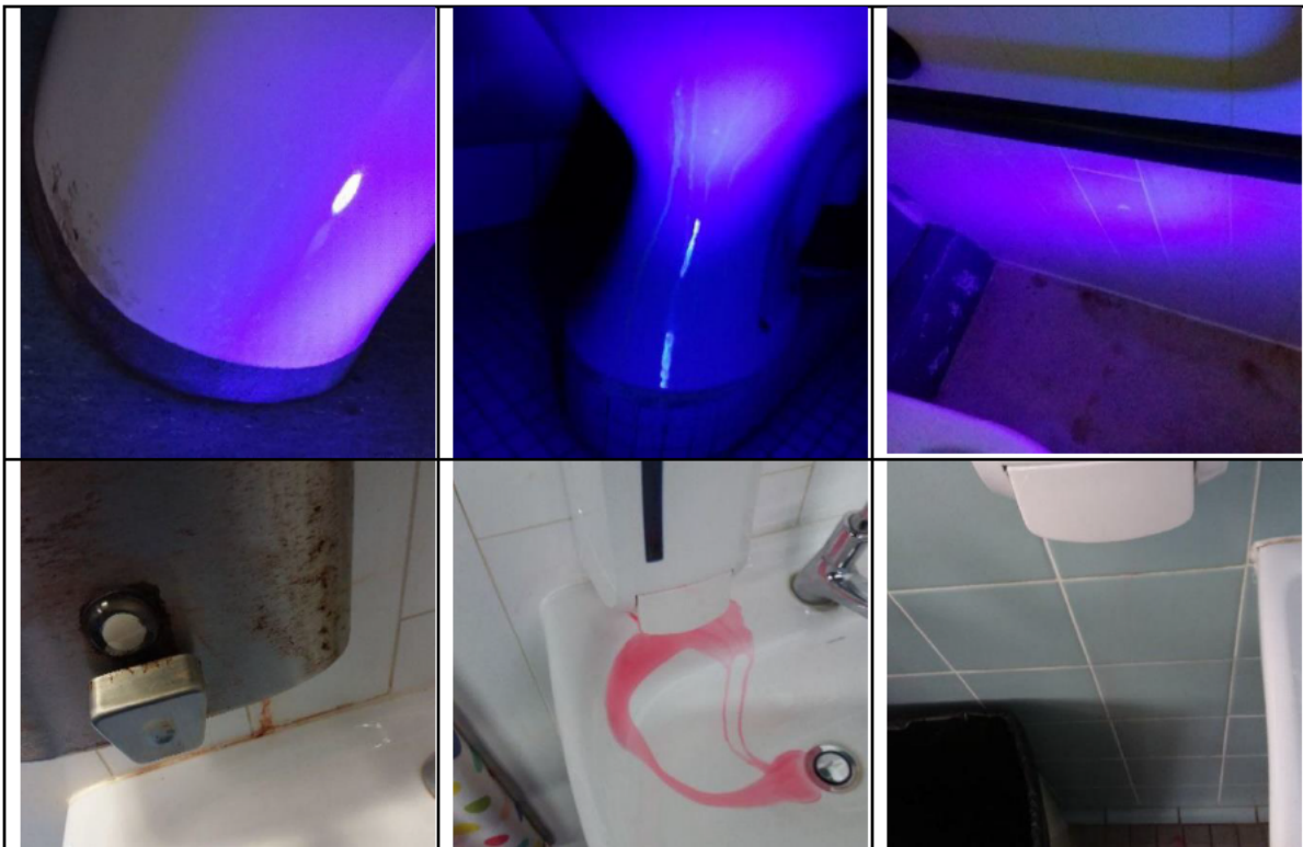
Figure 15: Top L-R: Urine runs and splash marks on toilet Cranleigh; Urine runs on Toilet - Malkara; Urine splashes on walls Malkara. Note soil on floor.
