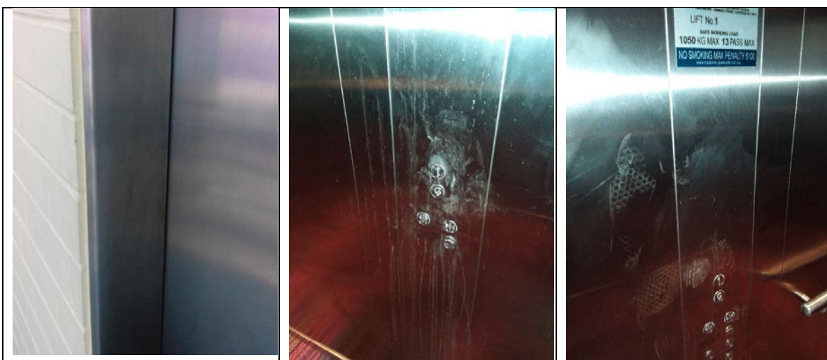
Figure 25: L-R: Lift Exterior doors Erindale College; Lift control panel and interior Harrison School (2 photos)
