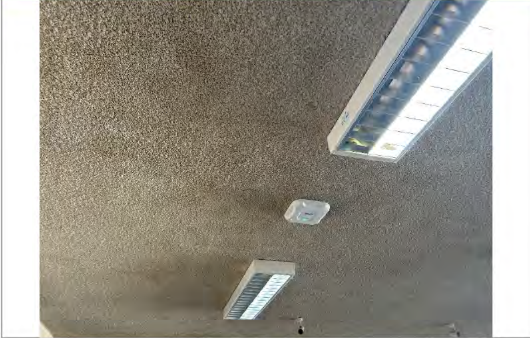
Photograph 1: Photograph following encapsulation
