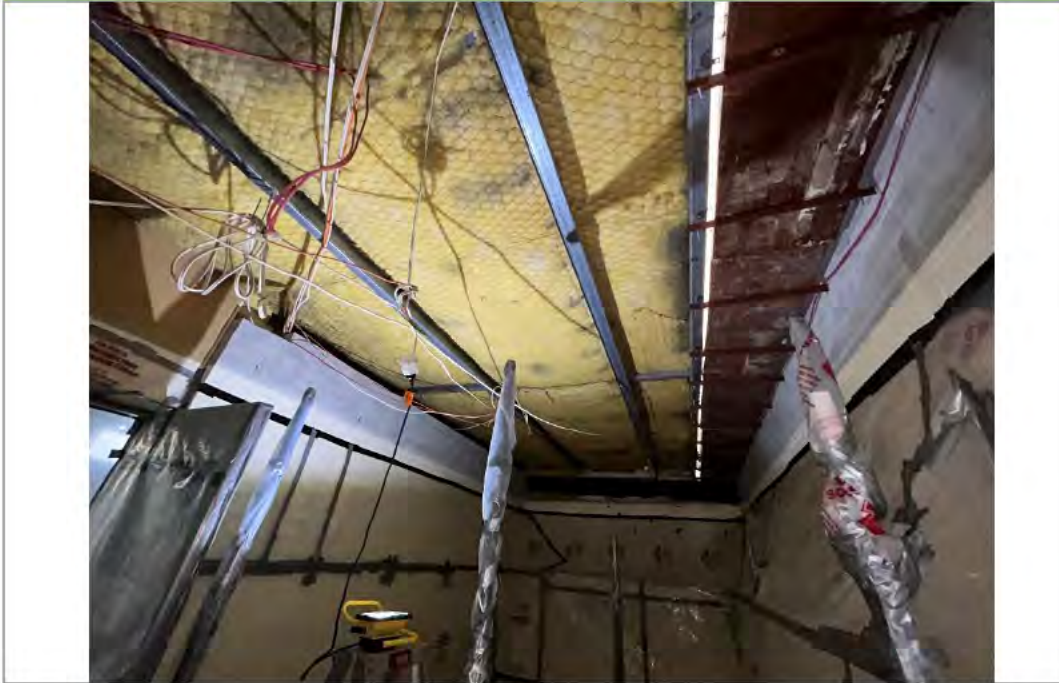
Photograph 1: Photograph following removal of asbestos spray coated ceiling
