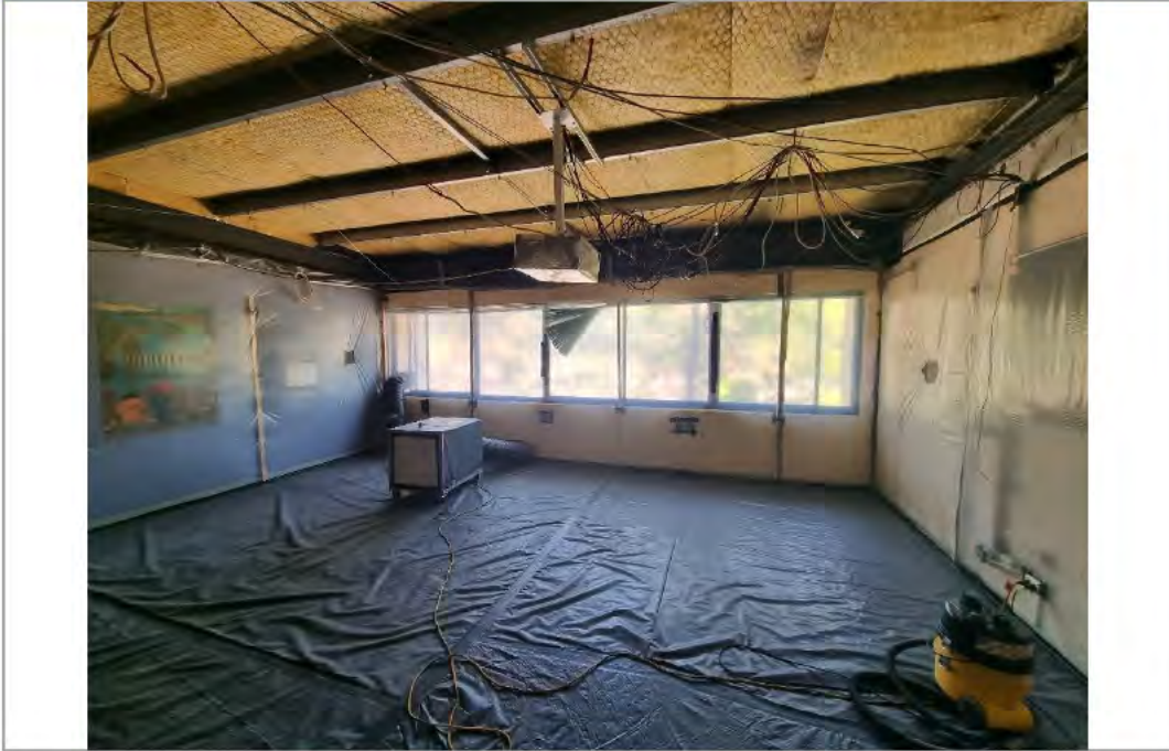
Photograph 1: Photograph following removal of asbestos spray coated ceiling from Room 7.4
