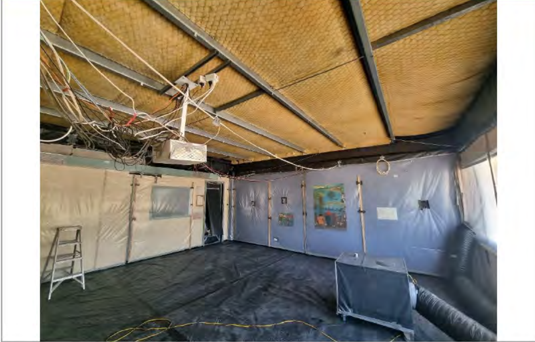
Photograph 3: Photograph following removal of asbestos spray coated ceiling from Room 7.4
