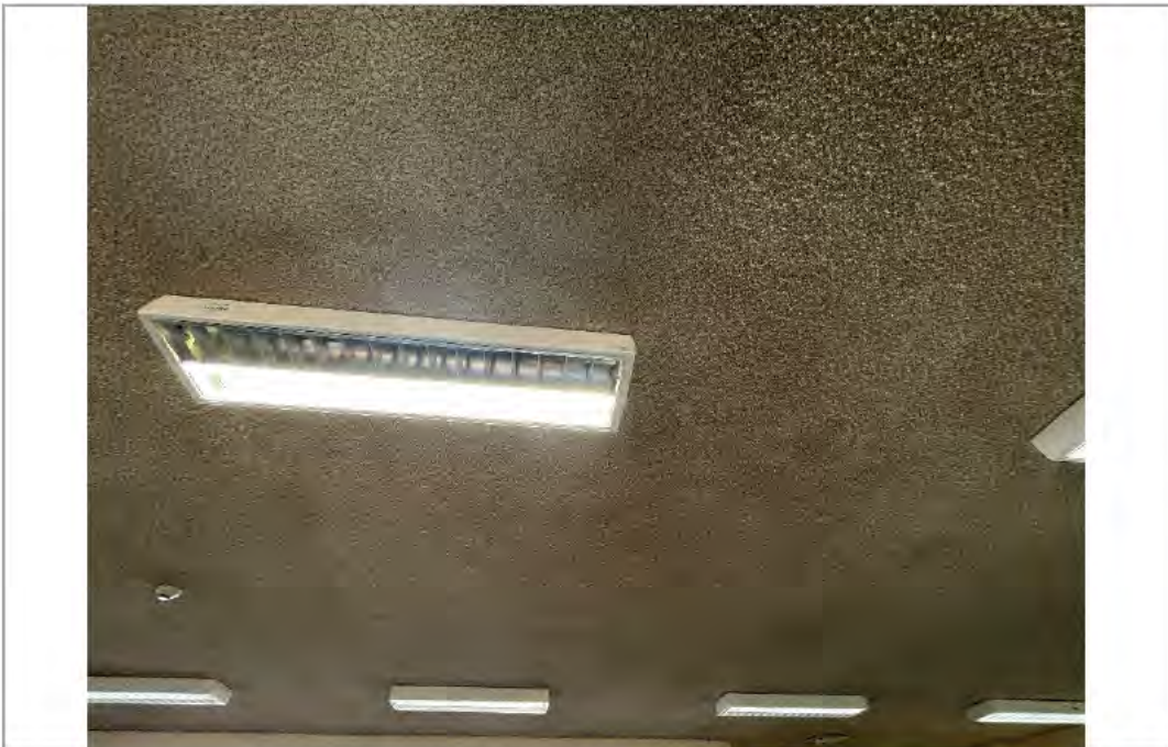
Photograph 1: Photograph following encapsulation
