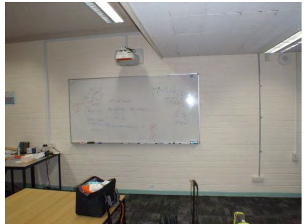
Figure 5 – L3122* - Masonry wall
