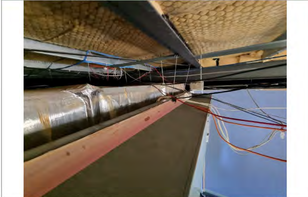
Photograph 5: Photograph following removal of asbestos spray coated ceiling from Room 7.4
