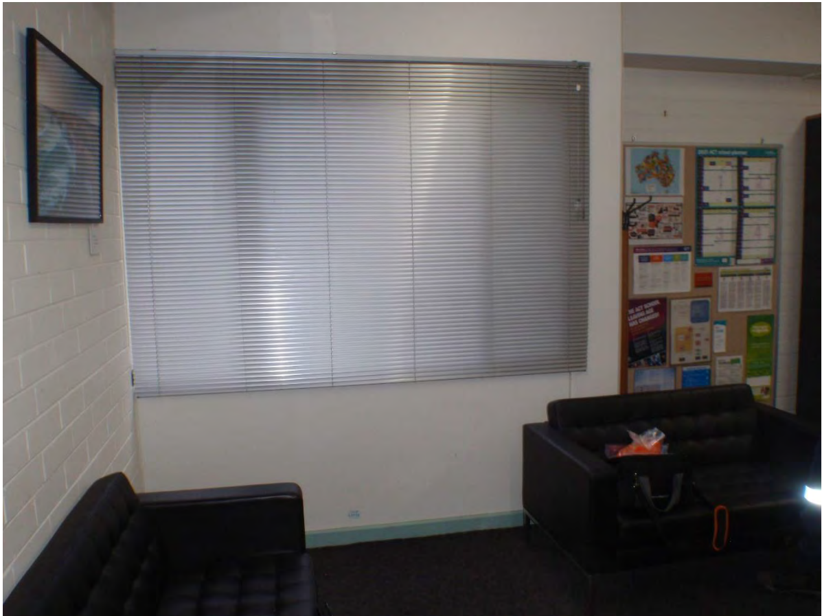
Figure 1 - L3119 - Masonry wall
