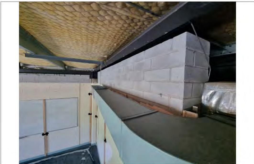
Photograph 4: Photograph following removal of asbestos spray coated ceiling from Room 7.4
