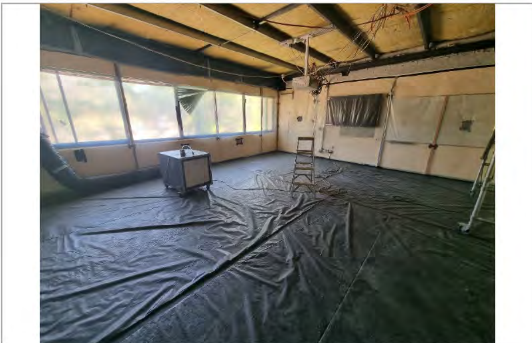
Photograph 2: Photograph following removal of asbestos spray coated ceiling from Room 7.4
