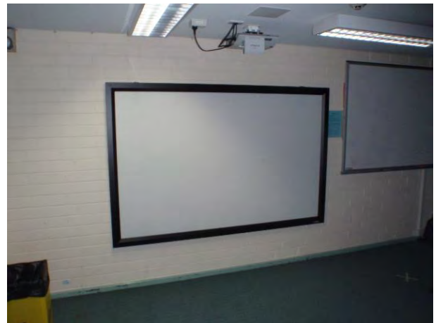
Figure 12 – L3130 – Masonry wall
