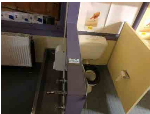
Figure 18: Sample W2266 top of partition
