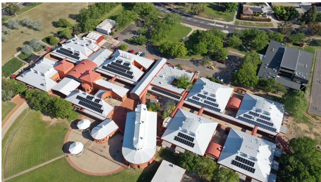
The solar expansion at Caroline Chisholm Senior School is paired with battery energy storage.
