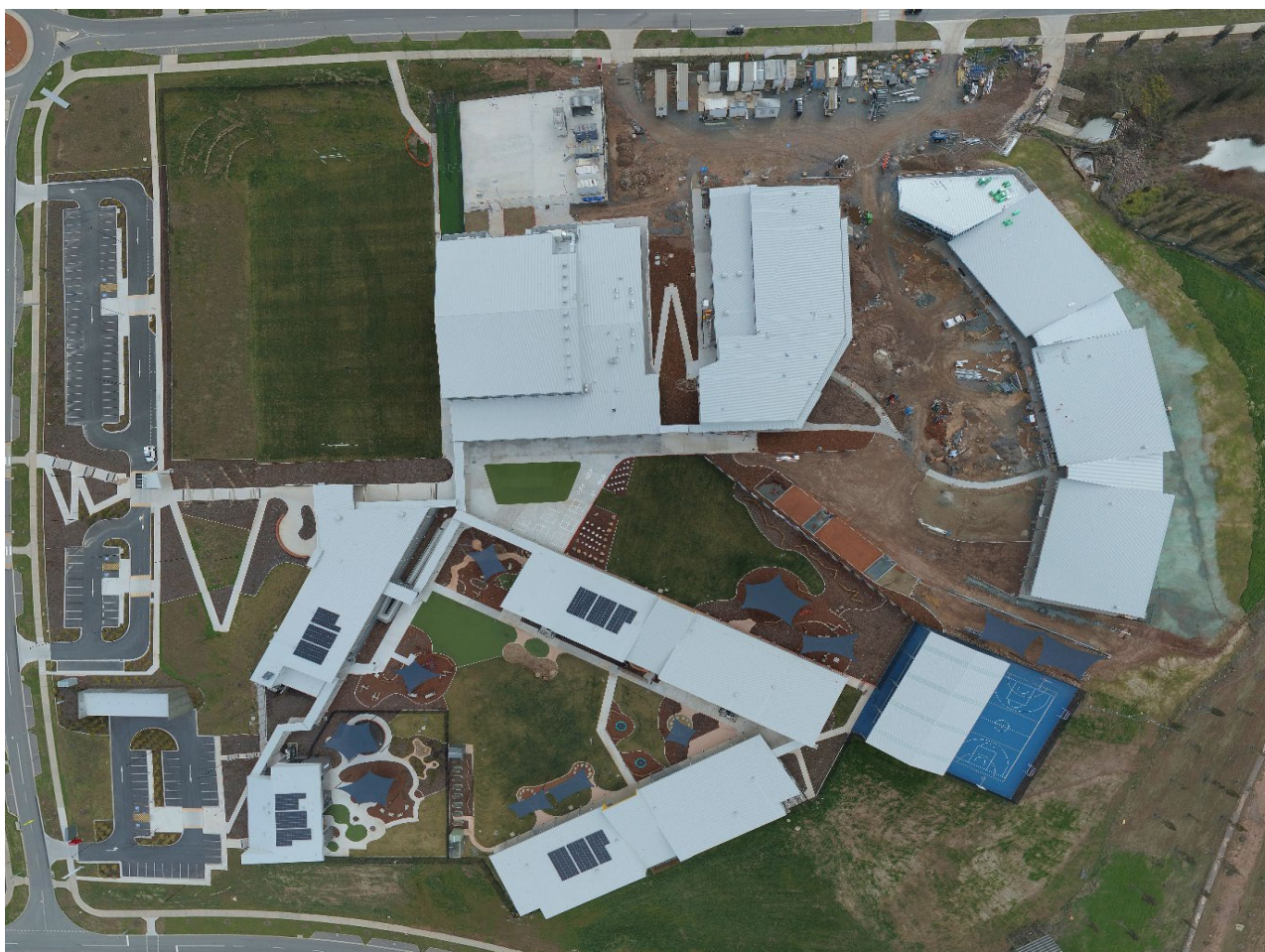
Drone image of Evelyn Scott School construction.
