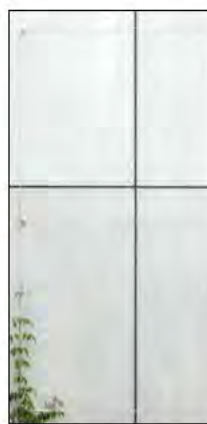
M.04 CEMINTEL BARESTONE EXTERNAL CLADDING COLOUR - CARESTONE
