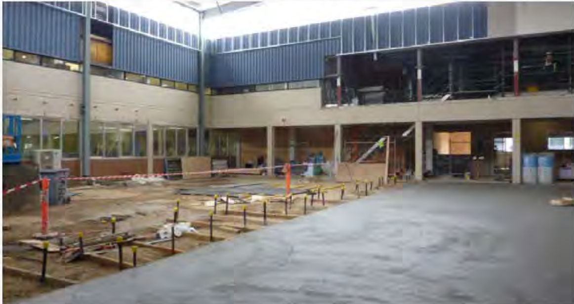
Belconnen High School - school modernisation project
