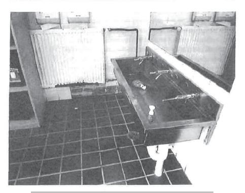
Above: exposed wall (asbestos?) where tiles have fallen off under broken, rusty and corroded heater.
