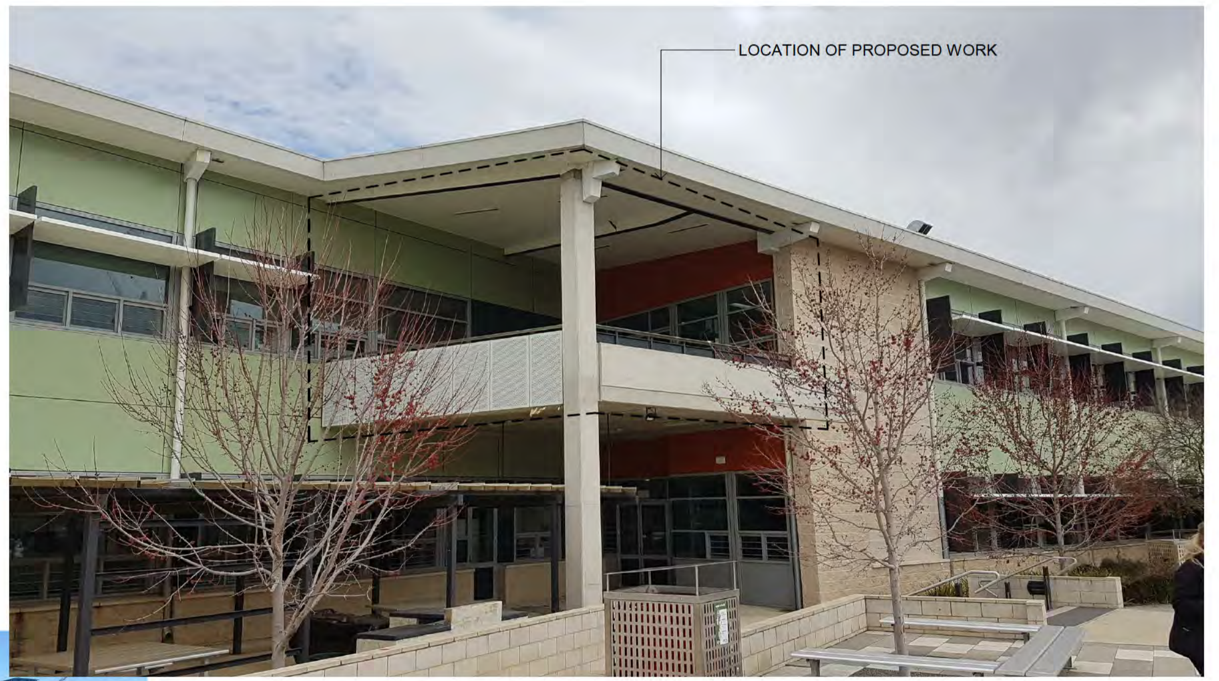
4 EXISTING WEST BALCONY PHOTO 1:50
