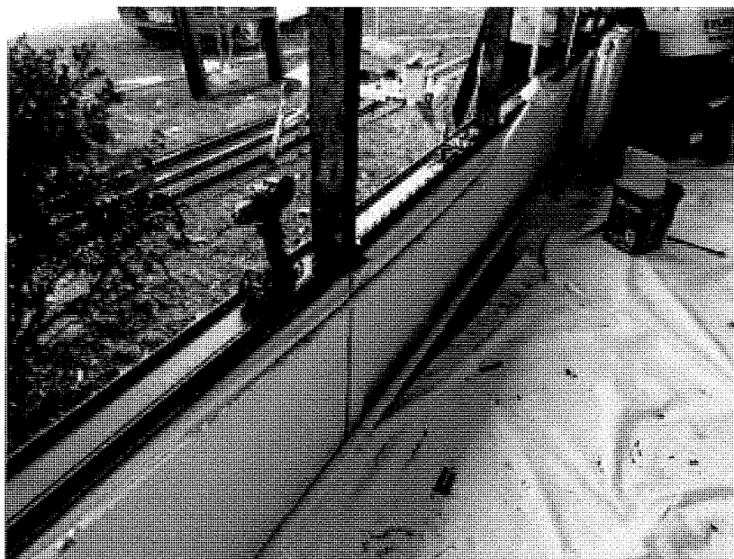
Figure 13: No exterior drop sheet
