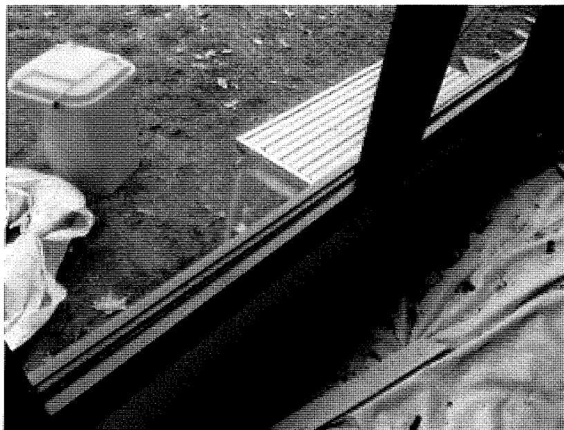
Figure 10: Inadequate drop sheets
