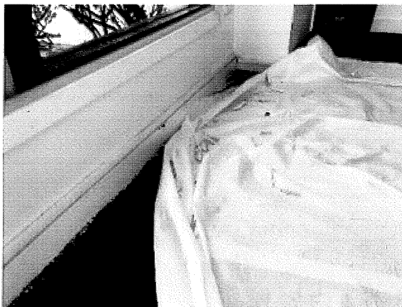
Figure 8: Ineffectual taping
