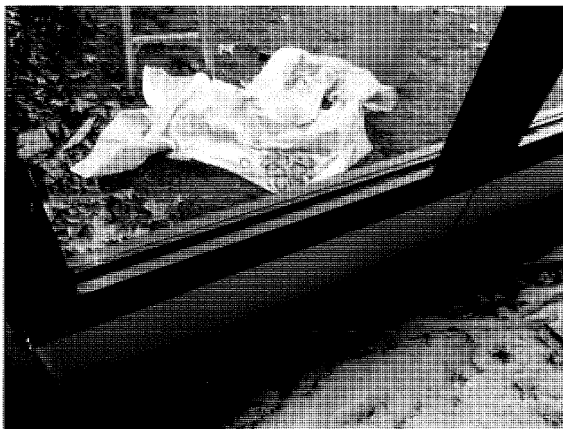
Figure 11: Inadequate drop sheets
